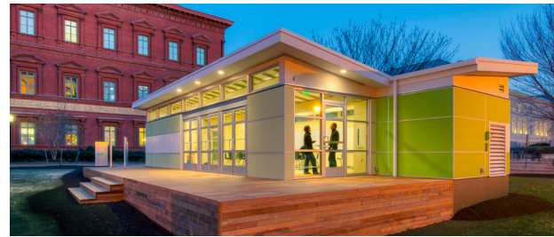
Figure 2: Sprout Space, TM a modular, single-room classroom system, as-built. This design concept was used as a starting point for material design exploration.
