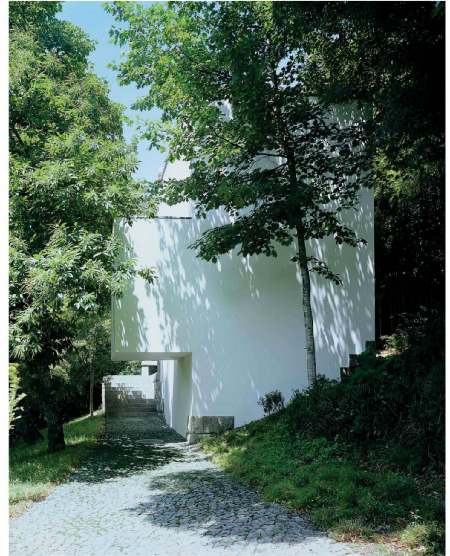
A simple chapel dedicated to St. Ovid was demolished under the instructions of a former owner. The new chapel, surrounded by vegetation, stands beside a coppice of linden trees at a high point on the site. The vestry space cantilevers out above the whitewashed chapel, forming the entrance porch to the sacred space, before the stairs that lead to the atrium.
